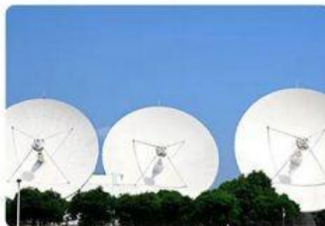
Communication base station monitoring power supply system
